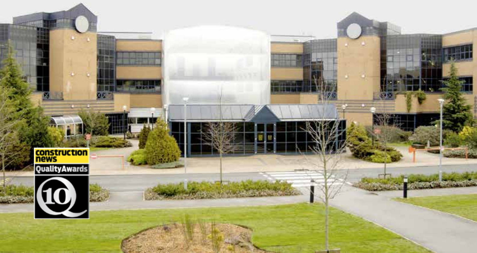
MBDA B100/200 office refurbishment, Stevenage - £10million
